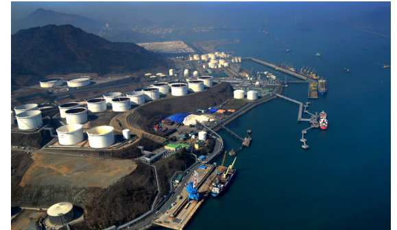
Yeosu tank terminal facility in Yeosu, South Korea
